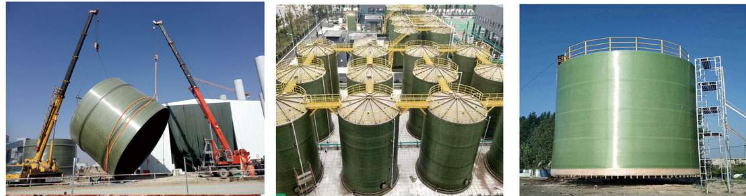
现场缠绕大型罐 SITE WINDING MAX TANK
